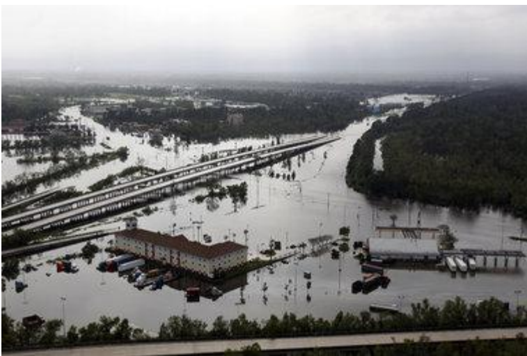
Hurricane protection at LaPlace was insufficient to keep
